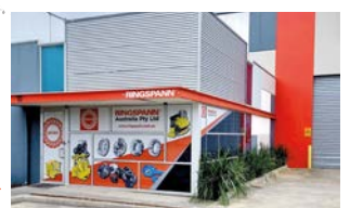
RINGSPANN Australia Pty Ltd., Australia
